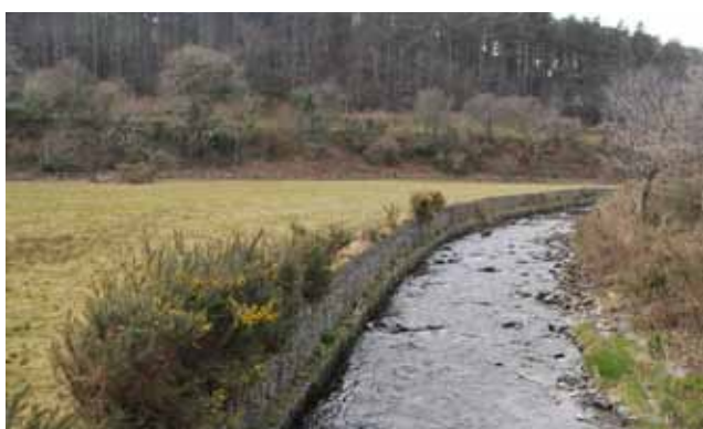
River bank protection © Martin Haslett
