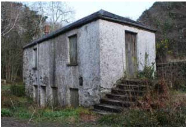
Ruined mine building © Martin Haslett
